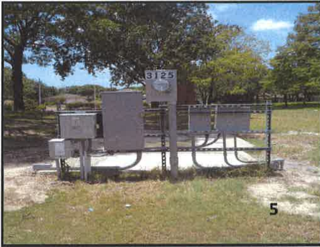
Completed Electrical Control Panel Replacement at Bundy Lake
