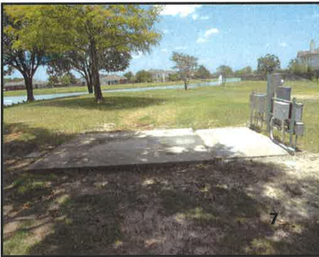
Bundy Lake Completed Vault Fill In and Seal
